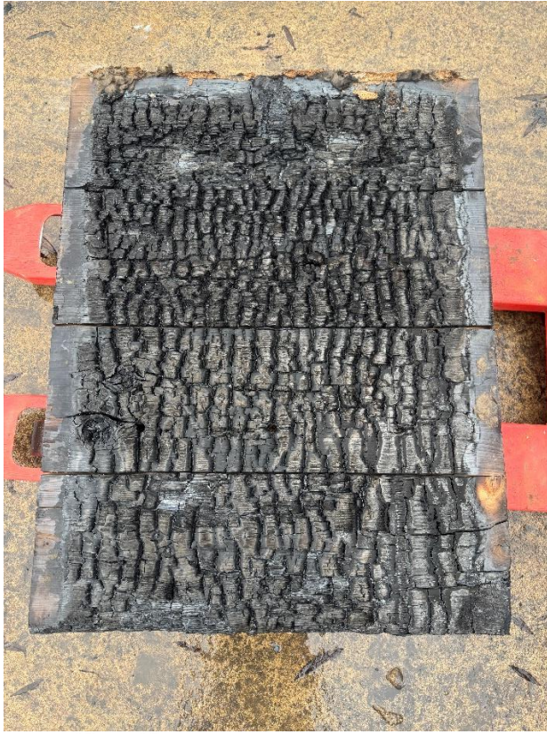
Figure 22 Ceiling panel post fire
