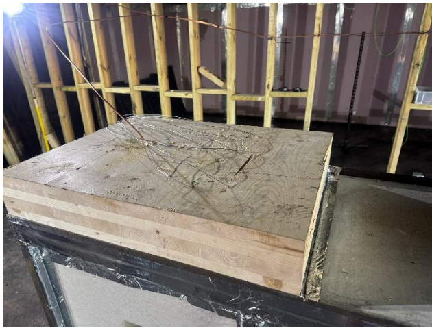
Figure 13 CLT ceiling panel
