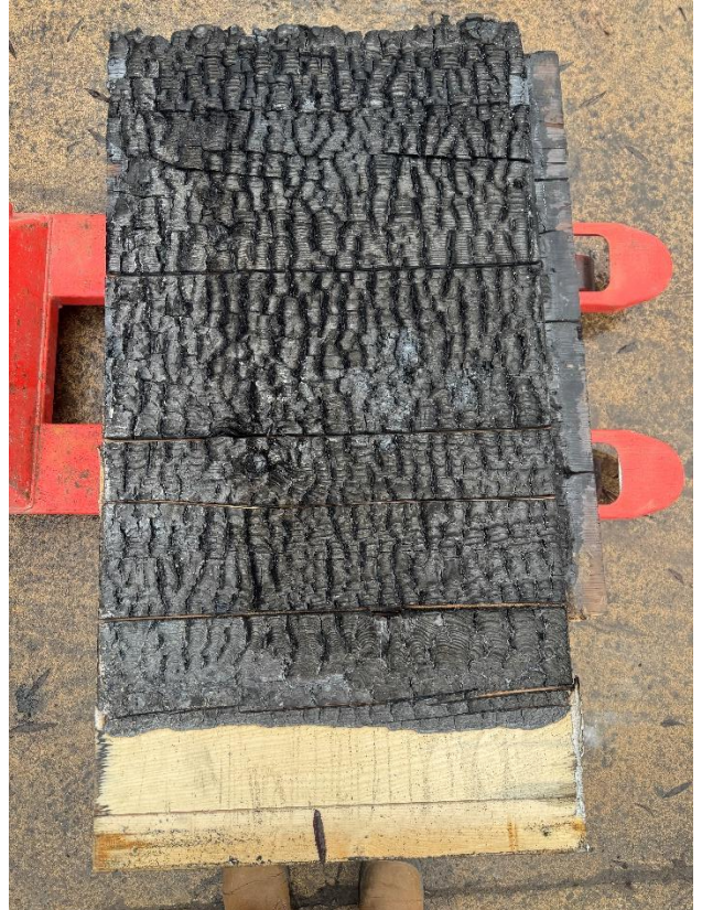
Figure 23 Wall panel post fire
