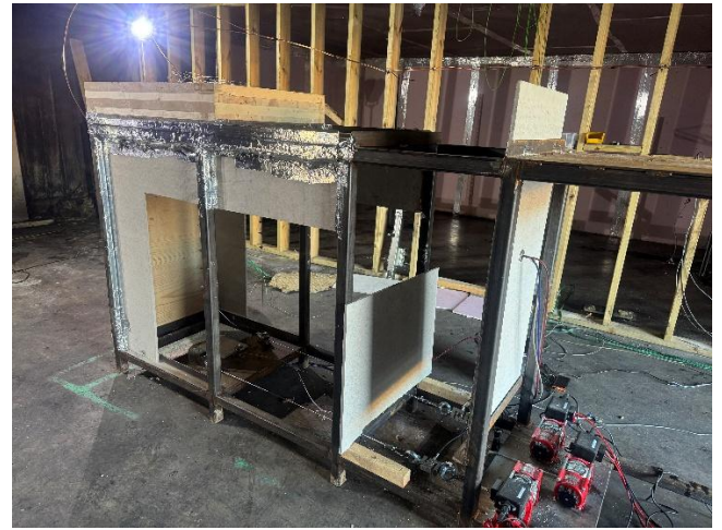
Figure 12 Side view of view with winch loading system installed
